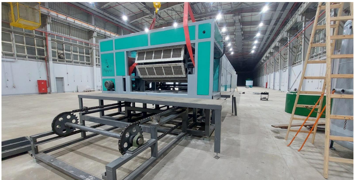
Figure 1: Installation of MP Moulding Line
